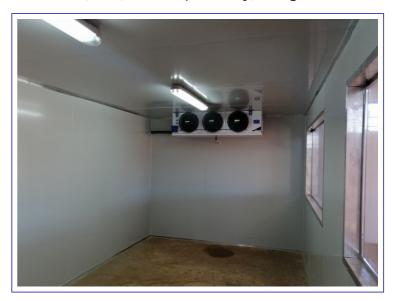
Refrigeration systems with scroll compressors are 15% to 20% more efficient than traditional reciprocating compressor systems. These compressors can be used for cooling milk or for space conditioning, such as a walk-in cooler. In addition to high-technology refrigeration equipment, a variety of supplemental refrigeration technologies are available to reduce energy costs. Well water-cooled plate heat exchangers can be used to pre-cool the milk before it enters the bulk tank.
